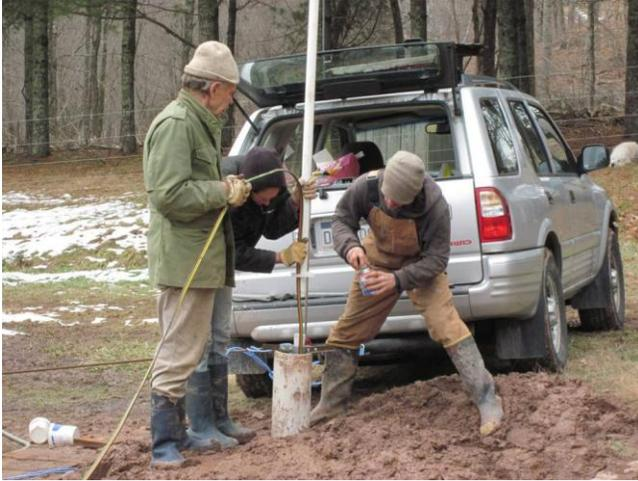
Step 2 - Pipe is vertical and requires slap guard. After the slap guard is on and wire in place, coat threads with sealant.
