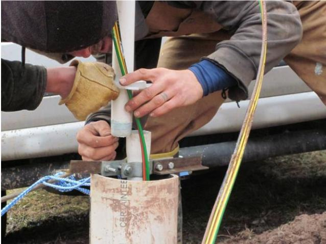
Step 2/3 - This is a nice view of the mechanism we used to clamp the pipe already in the well to the top of the casing so that we could thread the pieces together.
