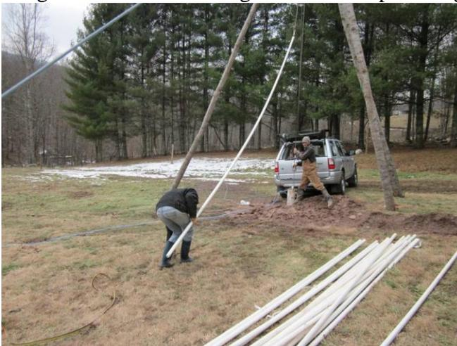
Step One - using a custom made plug with an eye bolt, we raise the stick of pipe above the casing of the well. Be careful not to bang the sticks around.
