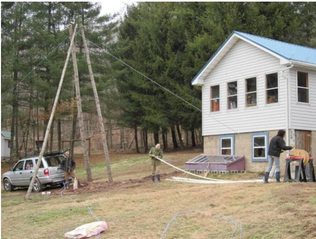
Overview of the project - note the gigantic tripod with pulley mounted on top, and the Isuzu being used as a counterweight. Yes the tripod has guy wires.
